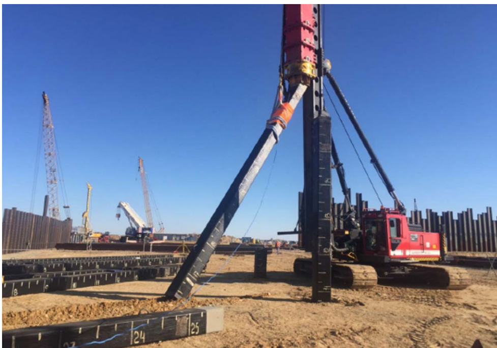
Figure 1 – Construction site of COF
