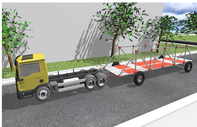
a) Overpass during transportation
