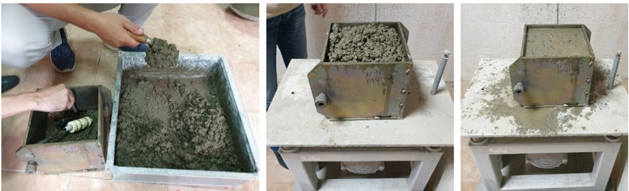
Figure 5 – Concrete pouring into the formwork and vibro-compacting
